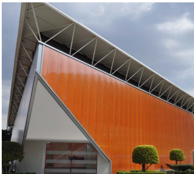
Cafeteria Unitec Atizapan, México | Vidro: Danpalon 3DLITE. Danpal 16 mm
